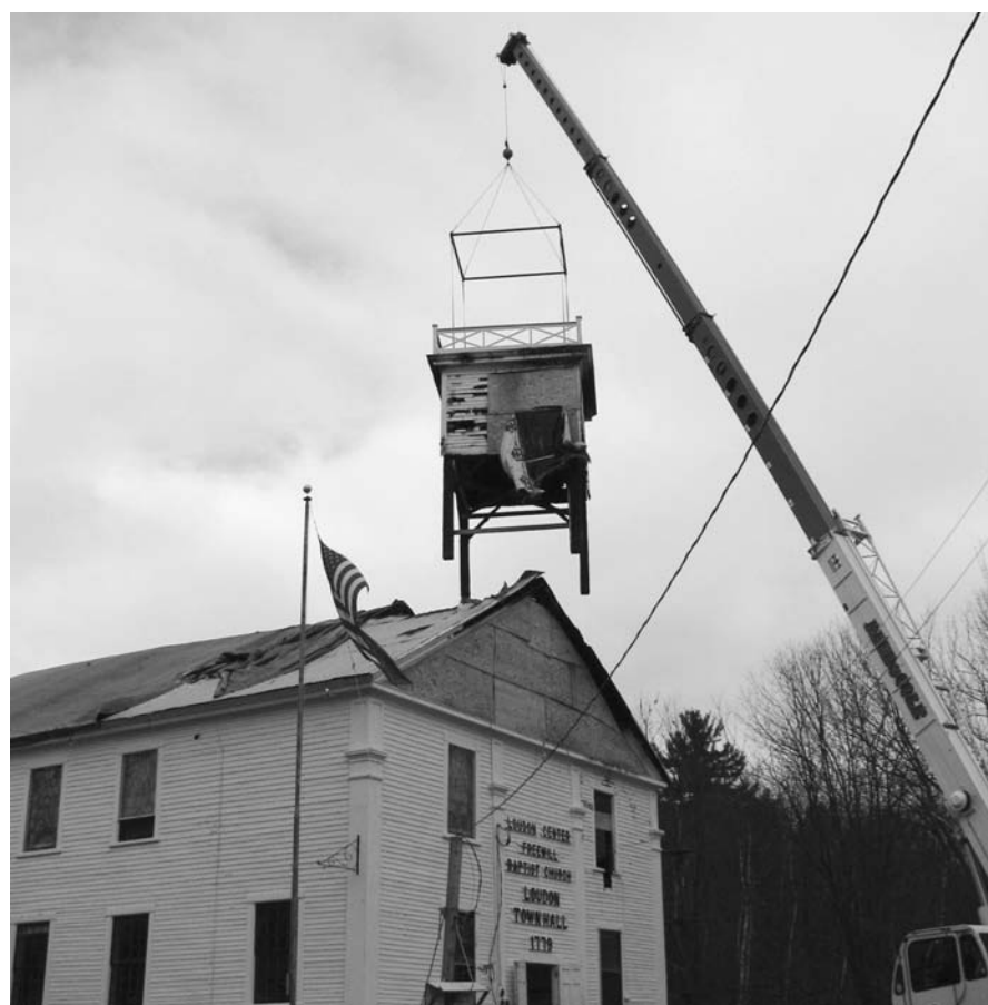
The steeple comes off so the roof can be replaced and the steeple repaired.
