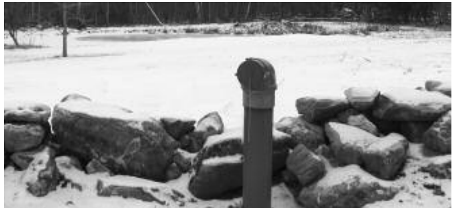
Above: The fire pond on property owned by Allan and Babbette Hanson, Bee Hole Road. Below: The dry hydrant connected to the pond. If you look carefully, you can see the pond in the background.
