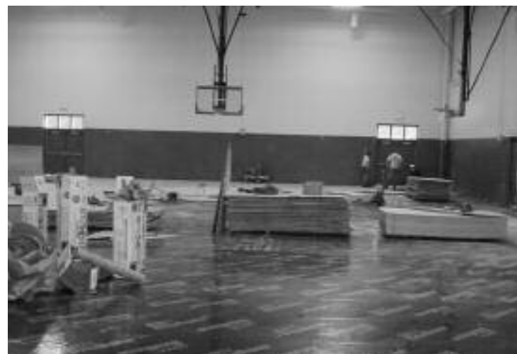
Sub-flooring being installed in the new gym.
