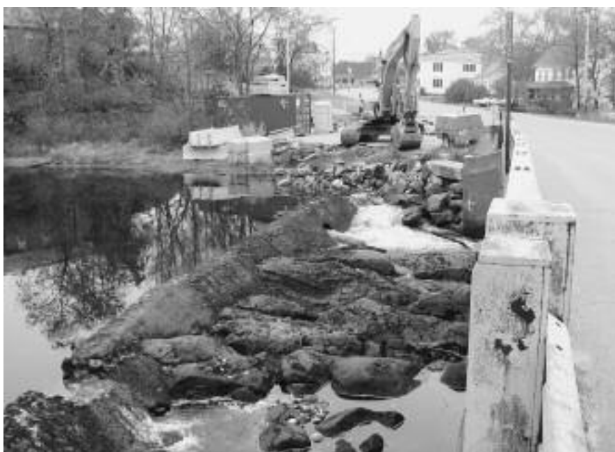
More May 2006 destruction undergoes repairs. The Mill Pond dam and banks were originally damaged in the Fall 2005 flooding and further worn away in May. Here, the pond is being drained so work can proceed.
