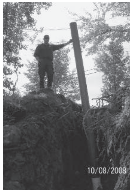
The top portion of the dry hydrant. John Reese shows how deep the hole is leading down to the bottom of the pond.
