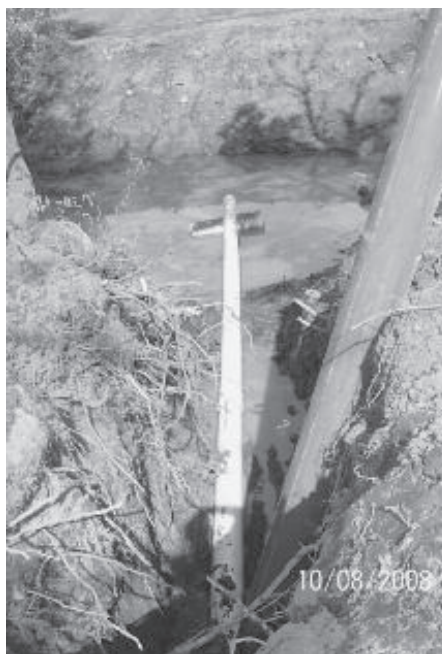
Looking down into the pond from the top of the dry hydrant.
