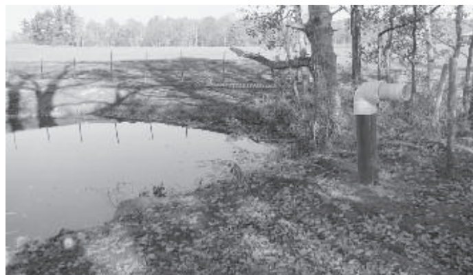
The finished pond, with the new dry hydrant, which is waiting for one last piece to arrive.
