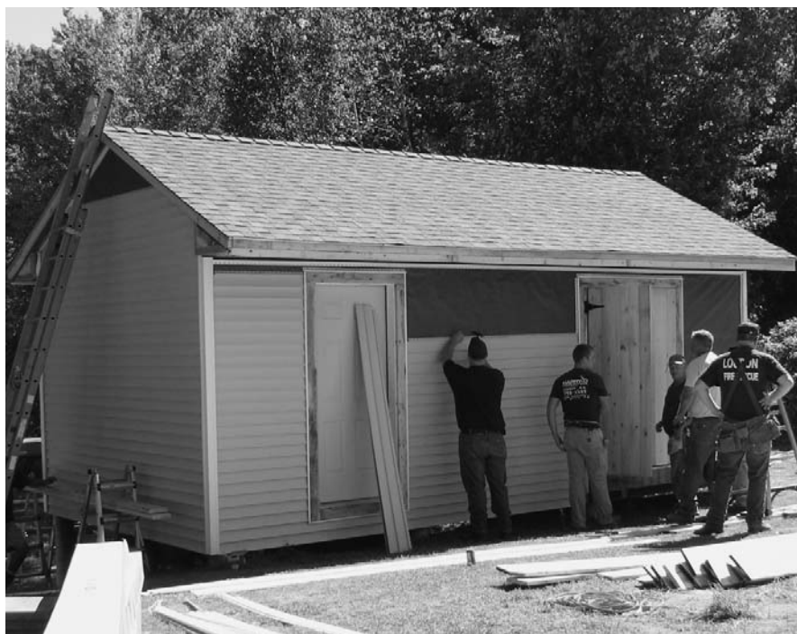
DAY 2: The siding is almost complete on the shed.
