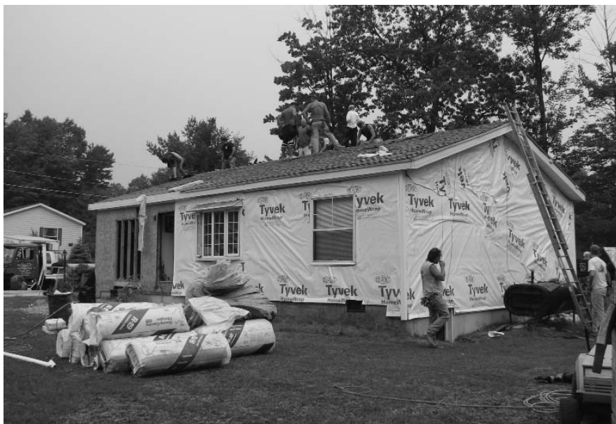
DAY 1: The house is wrapped and ready to put the siding on. Insulation awaits installation.
